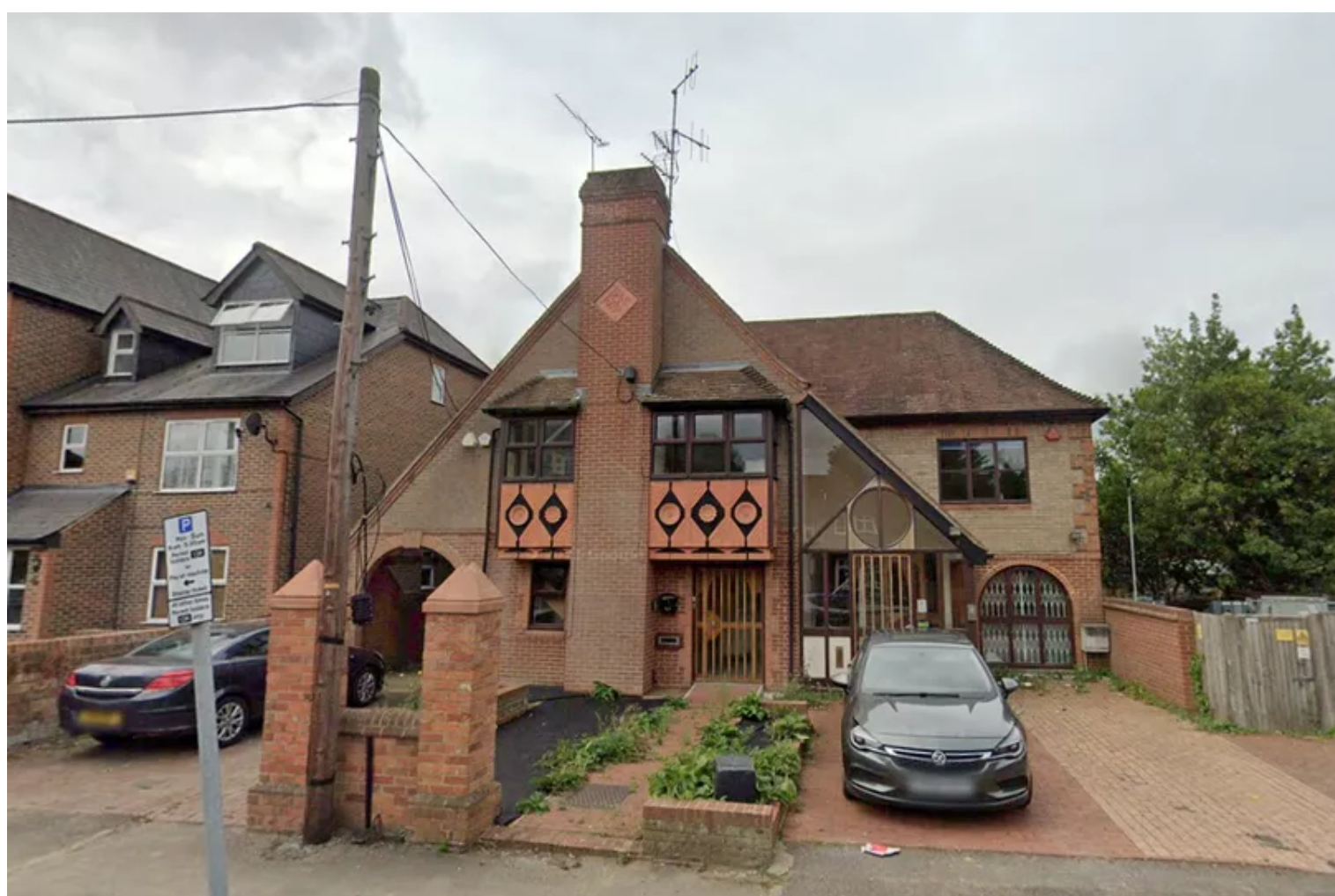
The current site has been vacant since 2019 (Image: Google Street View)
